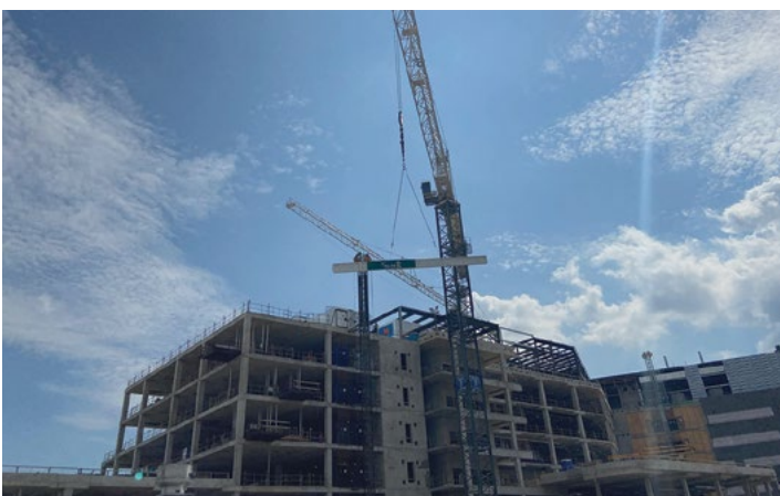
Final beam is lifted into place on roof of Outpatient Block
